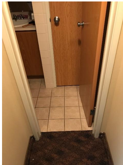
Figure 5.24. Brandon took this photograph of the door to his bathroom in his “handicap accessible” apartment.
