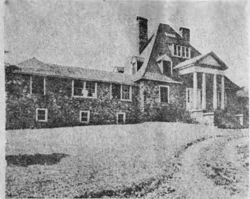
DOGWOODS, the main house on the homestead. One of the wings contains the workshop, the other the loom-room. Designed and built by amateur labor. Even the wiring, plumbing, and steam-fitting were done by what can at best be described as semi-skilled labor. The stonework in all the houses on Dogwoods was put in by amateurs, using a modification of the Flagg method of wall building.
